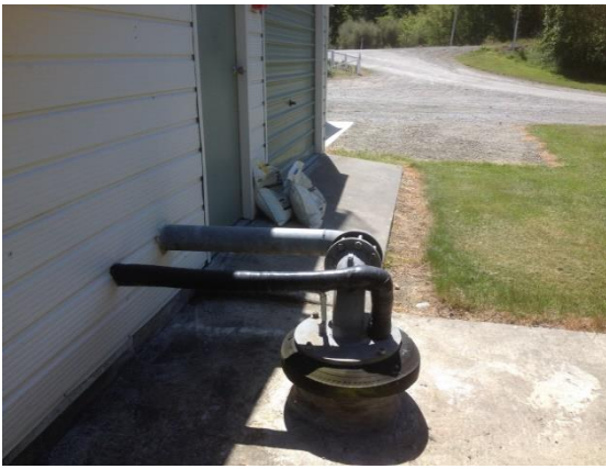
Photo 4 pipe protection between tanks
